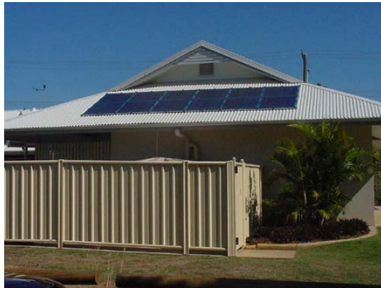
In the future perhaps every house will have a solar panel!
